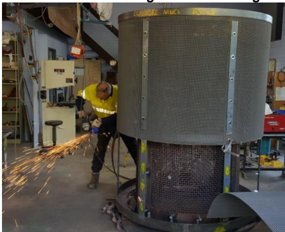
Fabrication of the sizing and de-watering screens
